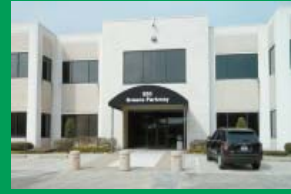
The Houston Intercontinental Chamber of Commerce has moved to 550 Greens Parkway, Suite 230 in Northeast Houston.
