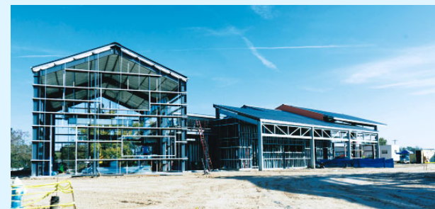
BakerRipley buildings well underway.
