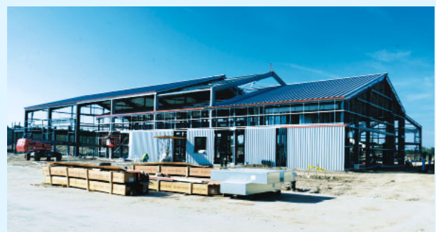
BakerRipley buildings receiving enclosing siding.
