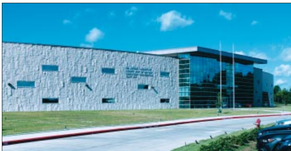
The Dr. Archie Blanson Career and Technical High School will be one of six new schools that will open in Aldine ISD when the 2018-19 school year begins on Monday, Aug. 20. The school is located at 311 West Road.
