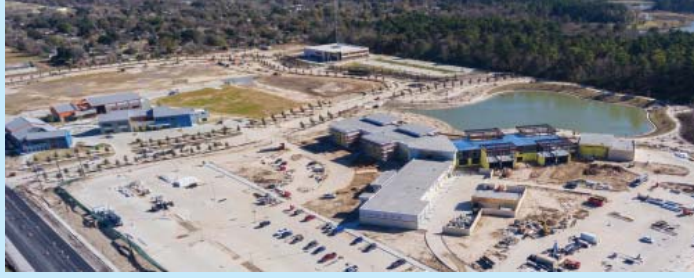
AERIAL VIEW FROM A DRONE shows the completed BakerRipley complex at the left, the Harris County 9-1-1 Call Center at the rear, and the Lone Star College-North Harris building at the right, under construction. (ev1 photo)
