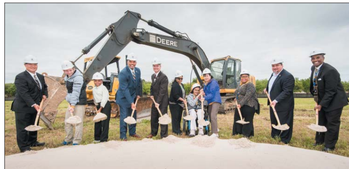
Harris County Department of Education Officials and community members at the groundbreaking of new Behavior School.
