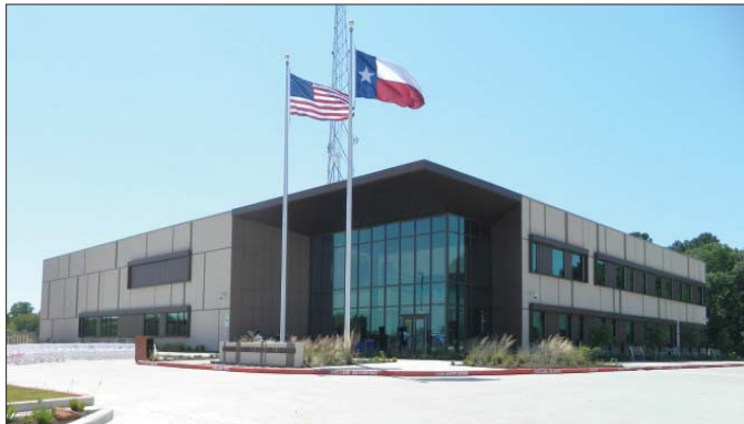
The New Harris County 9-1-1 Emergency Call Center is a two story, 42,000 square foot building, hardened to withstand hurricanes, floods, and other emergencies while its workers handle calls for help.
