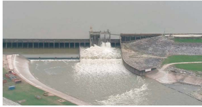
Lake Houston Dam will soon have new gates to help control flooding on the San Jacinto River watershed area.
