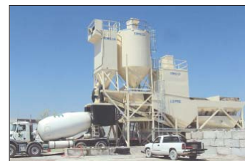
View of a typical Concrete Batch Plant
