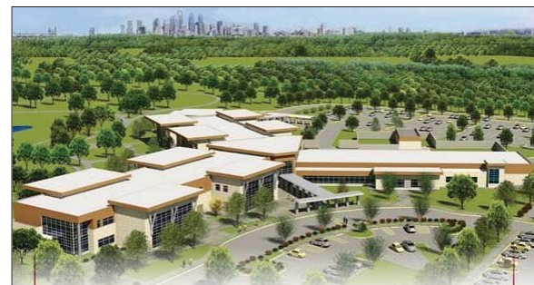
View of the new Lone Star College campus in East Aldine.
