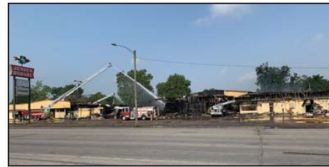
This scene along Jensen shows the complete destruction of several businesses, with Dollar General on the left, and the historic Granada Theater just out of sight on the right.
