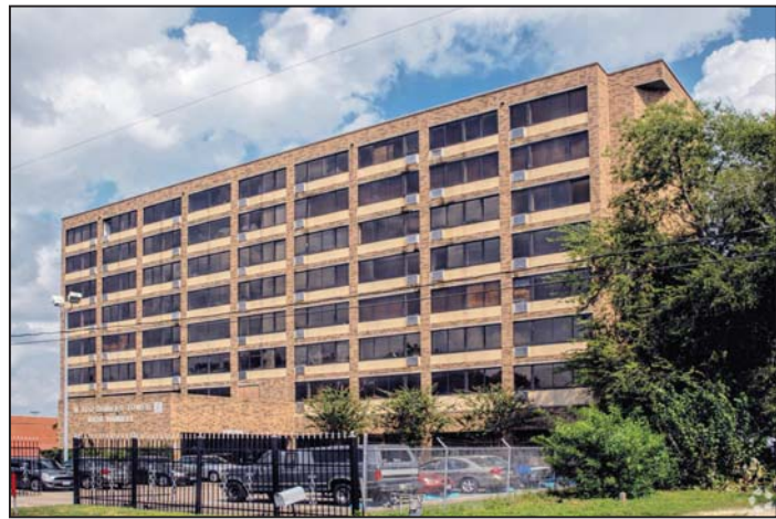
W. Leo Daniels Tower, named for a local pastor, was built over 40 years ago, and houses 100 apartments serving low rent elderly or disabled persons.
