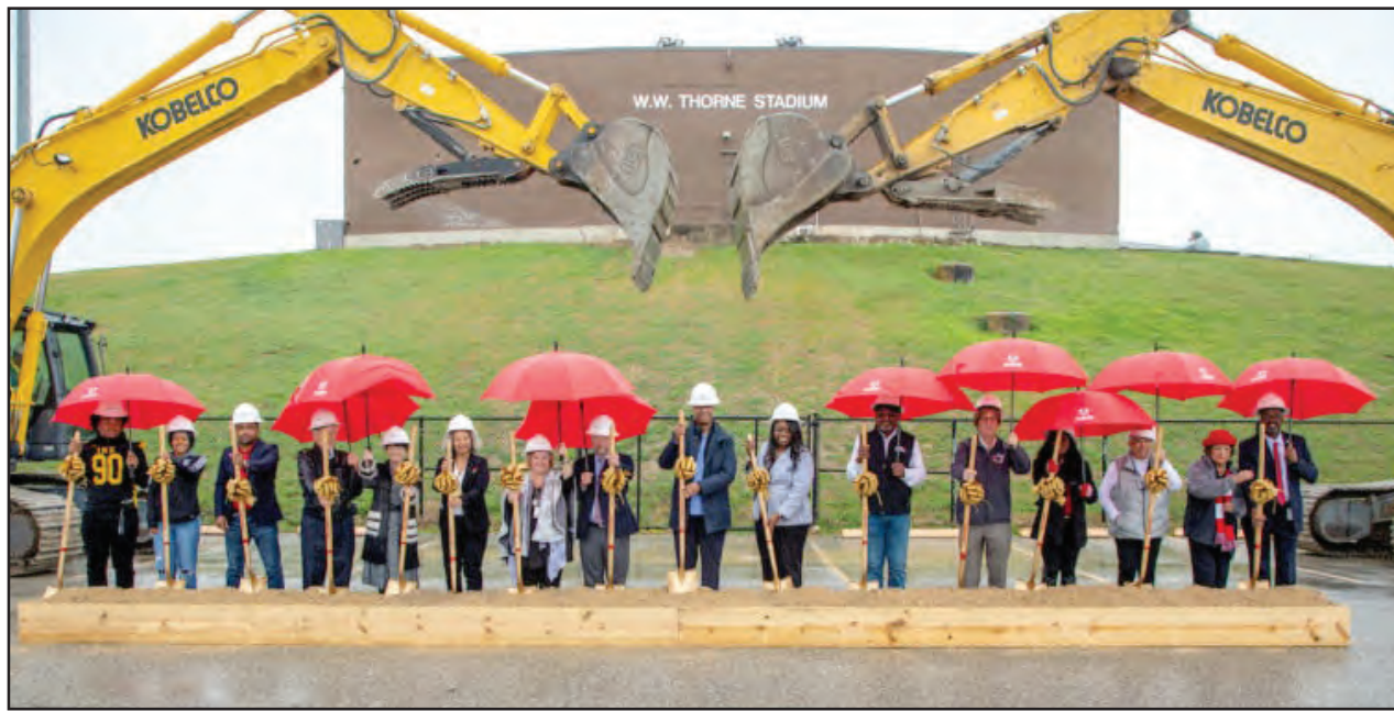
Groundbreaking for the new replacement W.W. Thorne Stadium was held Friday, January 20th in spite of heavy rain and wind. Administrators, athletic faculty, AISD board members, community members, students and Thorne family took part in the ceremony. Thoughtfully, somebody brought red umbrellas.
