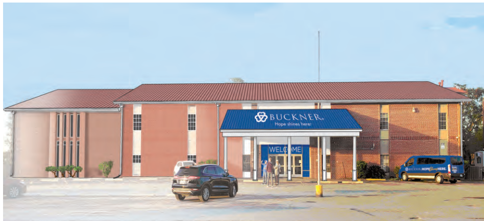
Buckner Family Hope Center will move from its location on Aldine Mail Route, to this building on Sweetwater Lane near I-45 North Freeway.
