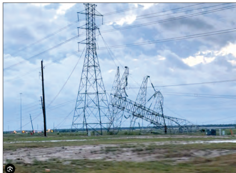
Transmission towers toppled by heavy winds, perhaps an EF-1 tornado, on the west side near Highway 99 and I-10.
