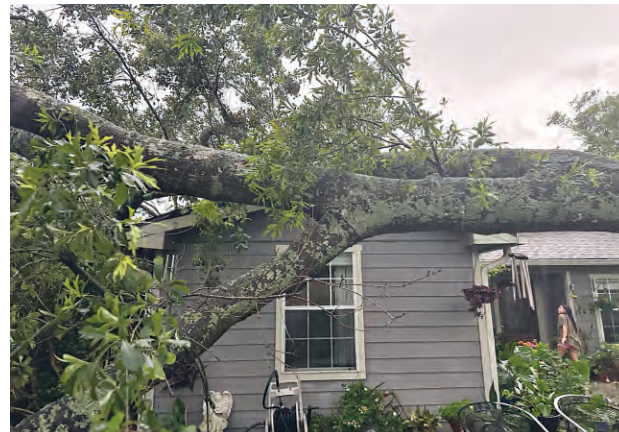
City wide destruction included fallen trees, flooded streets, downed power lines and transmission tower, and snarled traffic by accidents and traffic signals not working. This tree in the yard of a home in Garden Oaks is typical of hundreds throughout the city and the East Aldine District.
