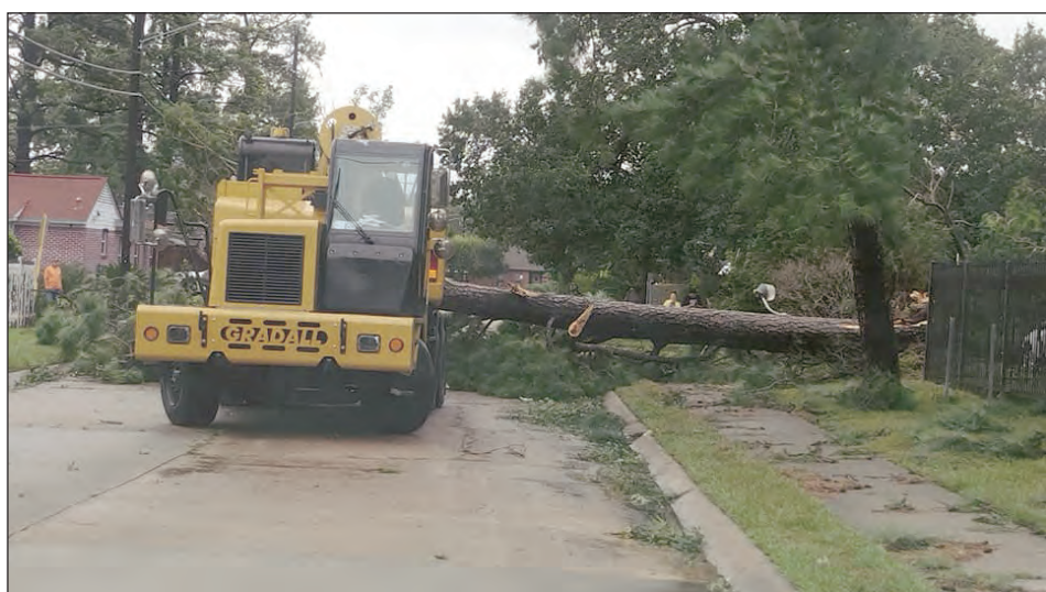
PCT. 2 CLEARS A FALLEN TREE WITH A GRADALL
