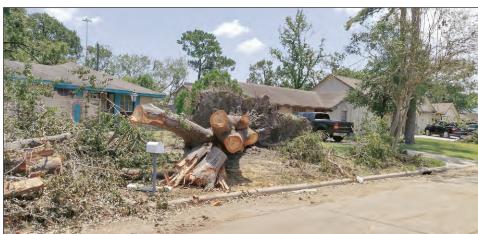
TREE ROOTS MUST STILL BE DISPOSED OF AFTER CUTTING AWAY THE TREE
