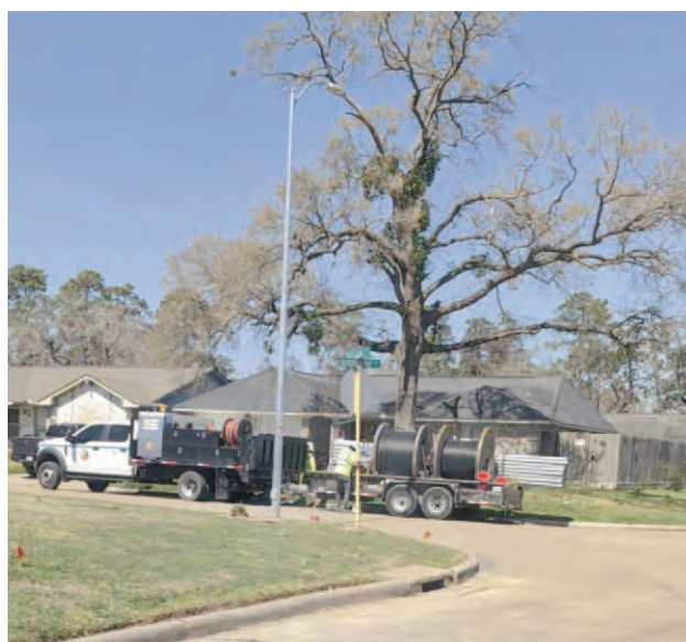
Electric Utility Crews installing poles and lights in HCWCID 74.
