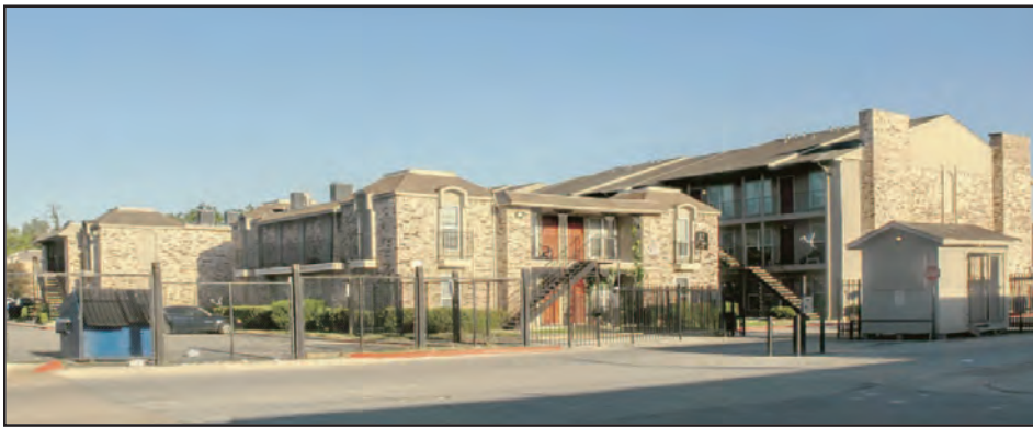
Haverstock Hills Apartments, a 700-unit affordable housing community in Houston's East Aldine, will be renovated by new owners.
